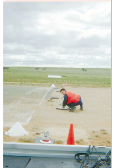
Fast deployment of AV70 threshold lights on 5kg non-slip tile
