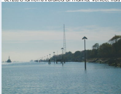
SL125/C lanterns installed at marina, Venice, Italy
